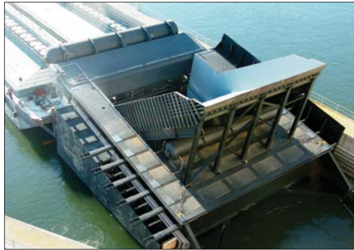
U.S. Army Corps of Engineers Photos
