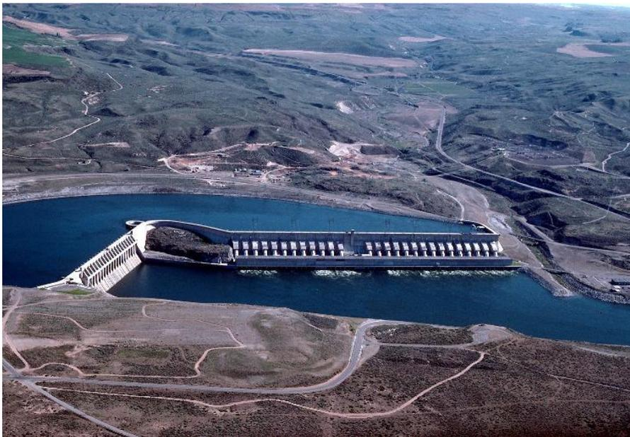
This modernization project will increase the facility's power generation capacity by more than 40 MW and boost turbine efficiency to 95% or better. Alstom's new ultra-efficient Francis runners (the central, rotating parts of hydroelectric turbines) are not only bringing the facility up to date, but when completed, will also deliver clean electricity to an additional 30,000 homes in the Northwestern U.S.
